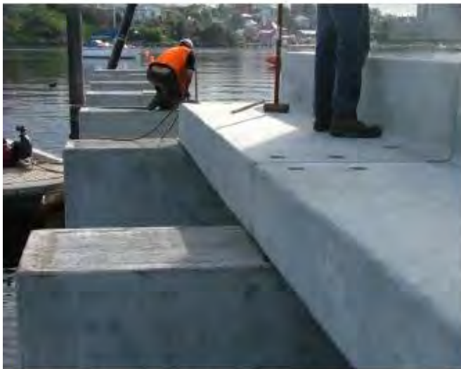
Photo C: View along pile caps showing fixed panels in place.
